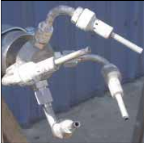
New spinner nozzles were installed at the locomotive wash.
