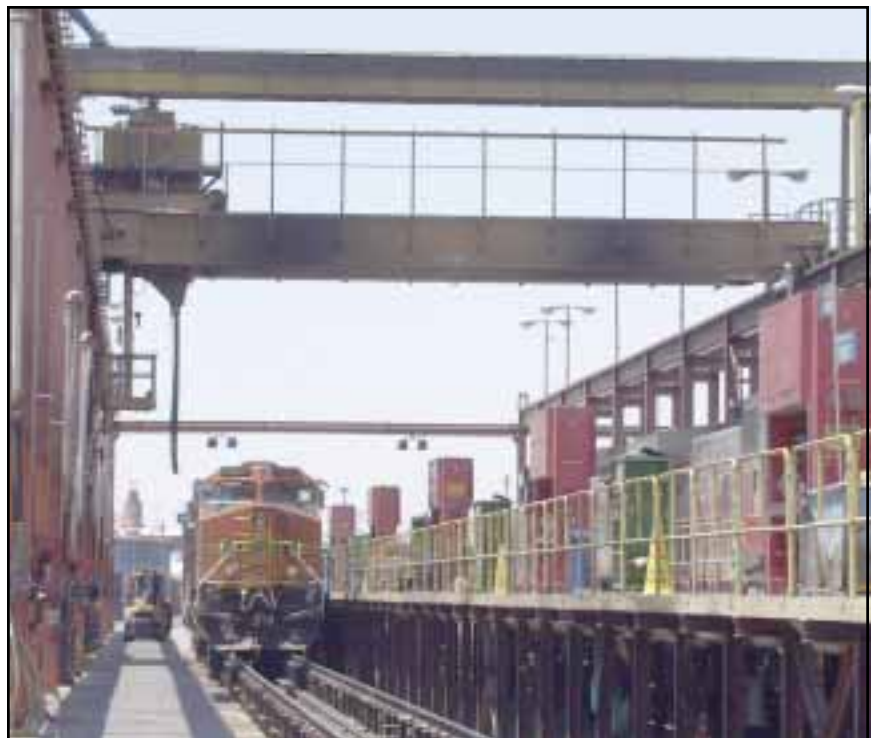
A 4-ton overhead crane will be installed on DSF tracks 14 and 15.
