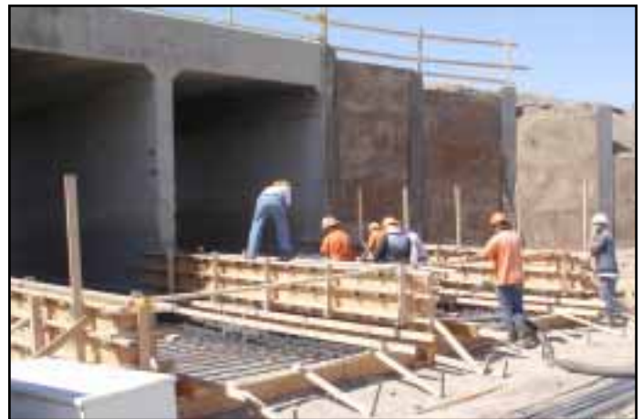
A system B&B gang readies forms for concrete.
