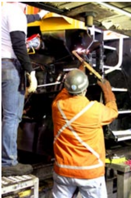
Dave White makes the final welds to repair 6090.
